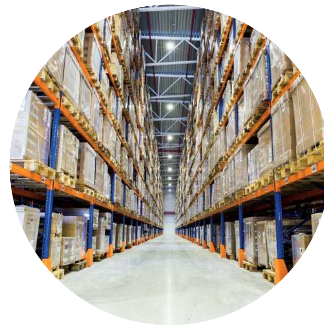
STORAGE & DISTRIBUTION SERVICES
